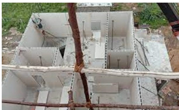
Figure 81: Glass Fiber Reinforced Gypsum (GFRG) panels for creating thermally insulated partition walls
