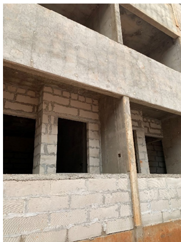
Figure 80: Use of AAC blocks (fly ash based) in partition wall of EPC model
